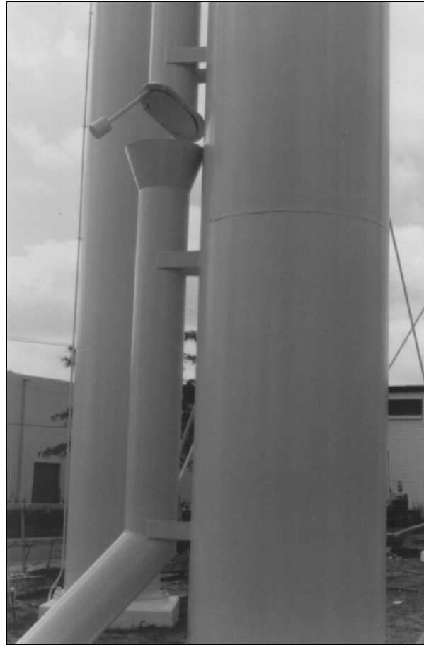
Figure 2-5 Overflow air break with flap valve
