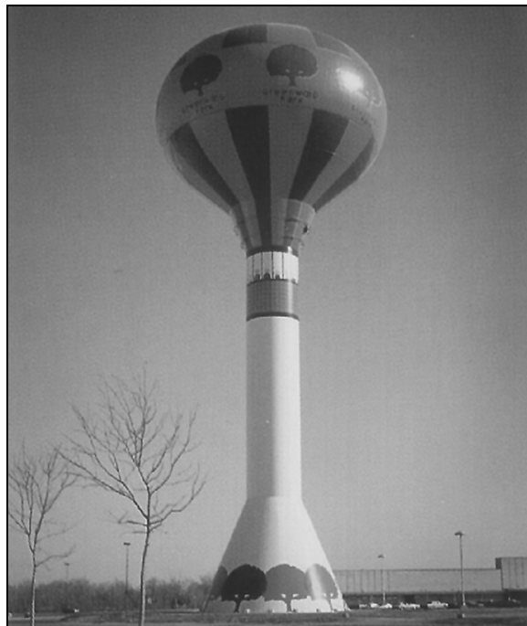
Figure 1-22 Large-capacity single-pedestal elevated tank
