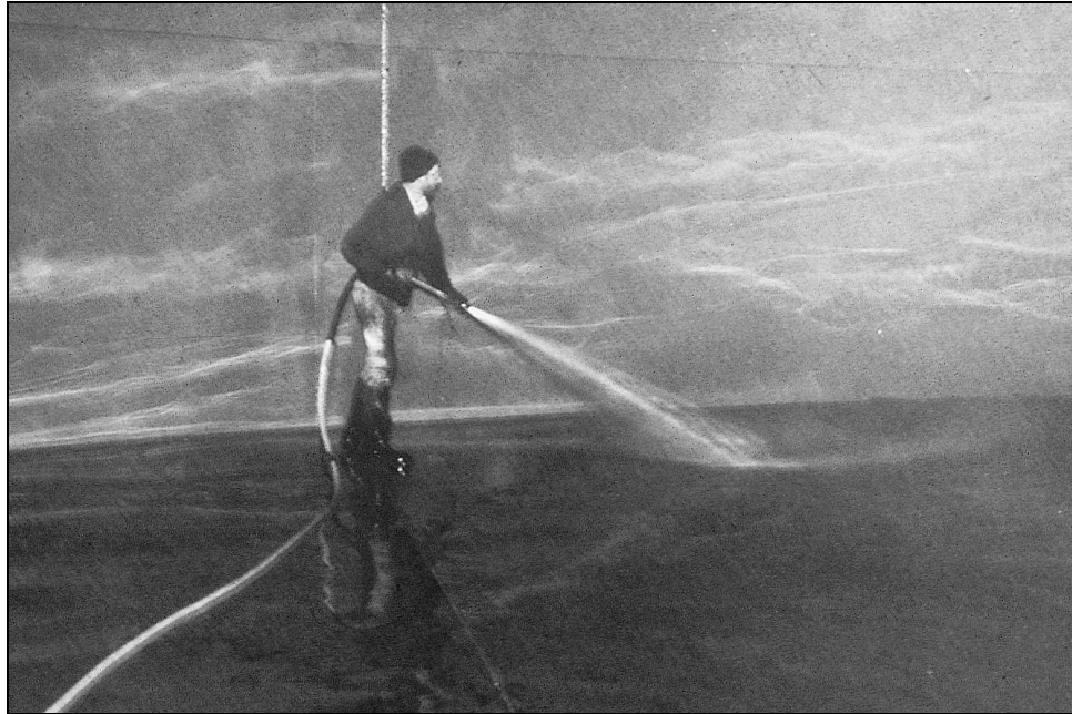
Figure 9-4 Washing out tanks allows easier inspection and keeps tanks sanitary
