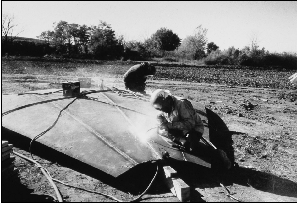
Figure 7-2 Typical welding operation in the field
