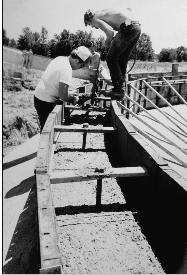
Figure 7-1 Tank foundation construction
