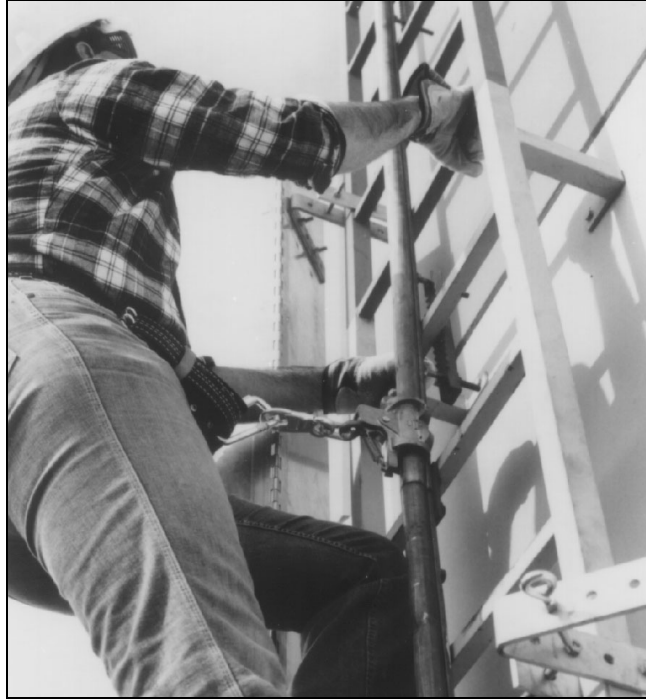
Figure 2-7 Safe-climbing rail for an outside ladder
