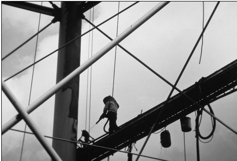
Figure 9-6 An abrasive blast-cleaning operation
