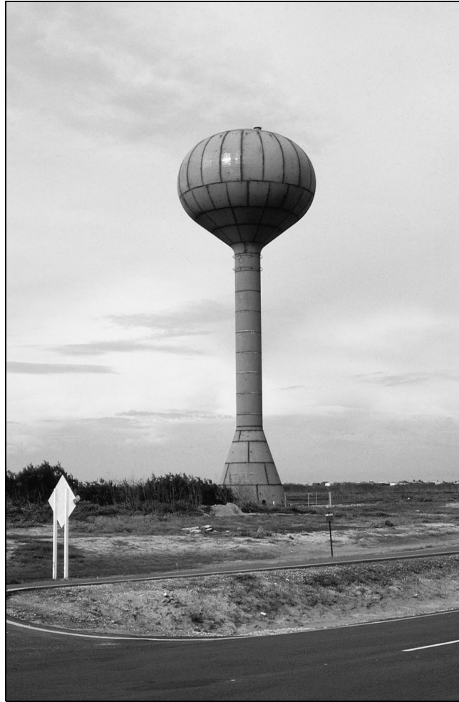
Figure 7-4 Newly erected elevated tank
