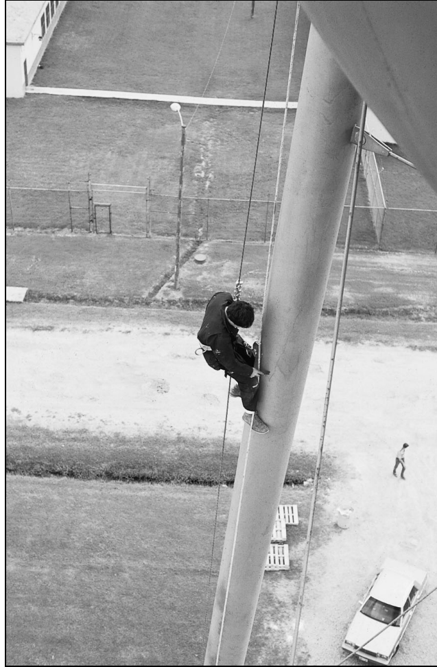
Figure 9-1 Experienced riggers evaluate hard-to-reach areas on tower tanks
