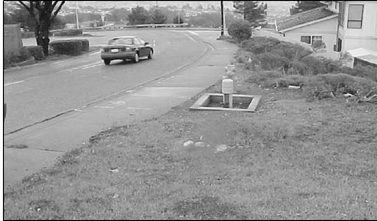
Figure 8-16 Programmable blow-off next to a hydrant used to flush dead-end to increase residual
