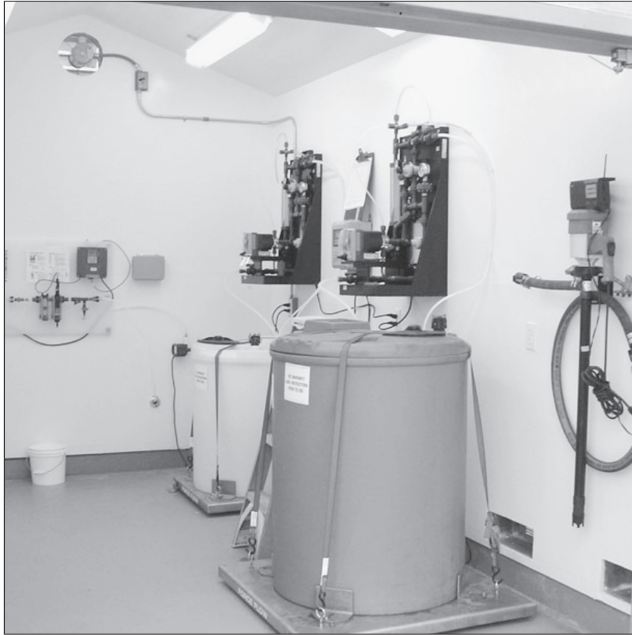
Figure 8-5 Sodium hypochlorite and liquid ammonia feed system at a wellhead where chlorine is added first
