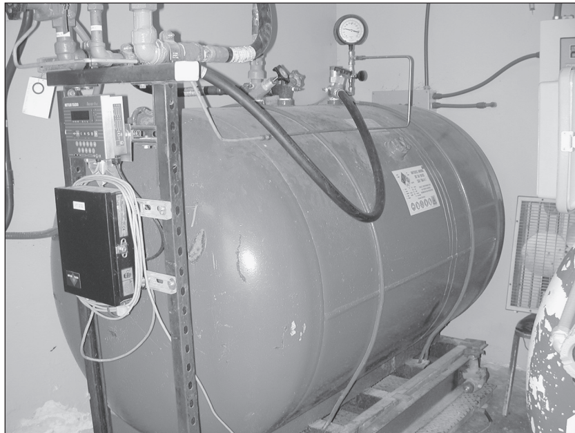
Figure 8-4 Example of an anhydrous ammonia feed system
