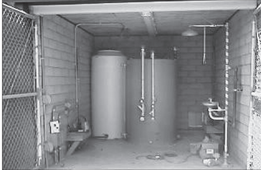
Figure 8-3 Example of an aqua ammonia (ammonium hydroxide) 500-gal storage tank and metering pump
